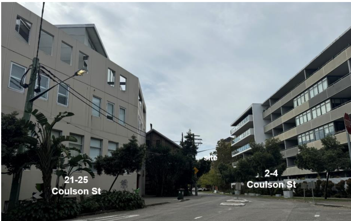
Figure 10: Neighbouring property at 21-25 Coulson Street and 2-4 Coulson Street
