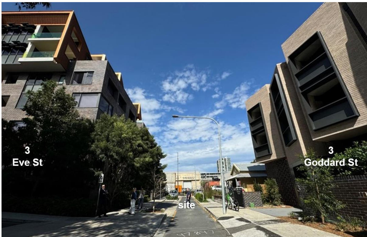
Figure 3: Site (7-19 Coulson Street) viewed from Goddard Street, with neighbouring property 1-3 Goddard Street and 3 Eve Street
