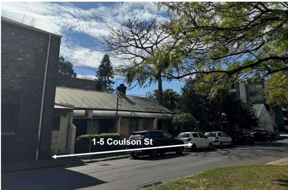
Figure 14: Neighbouring property at 1-5 Coulson Street
